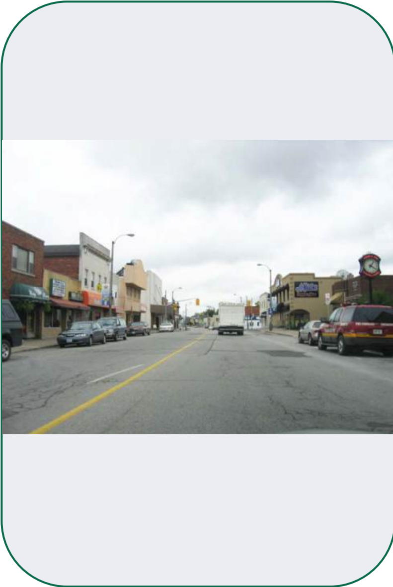
Figure 7.4 – Existing Main Street Streetscape
