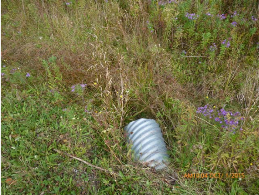
Photo 13: Culvert inlet in good condition.
