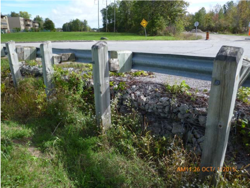
Photo 29: Gabion baskets supporting road surface.
