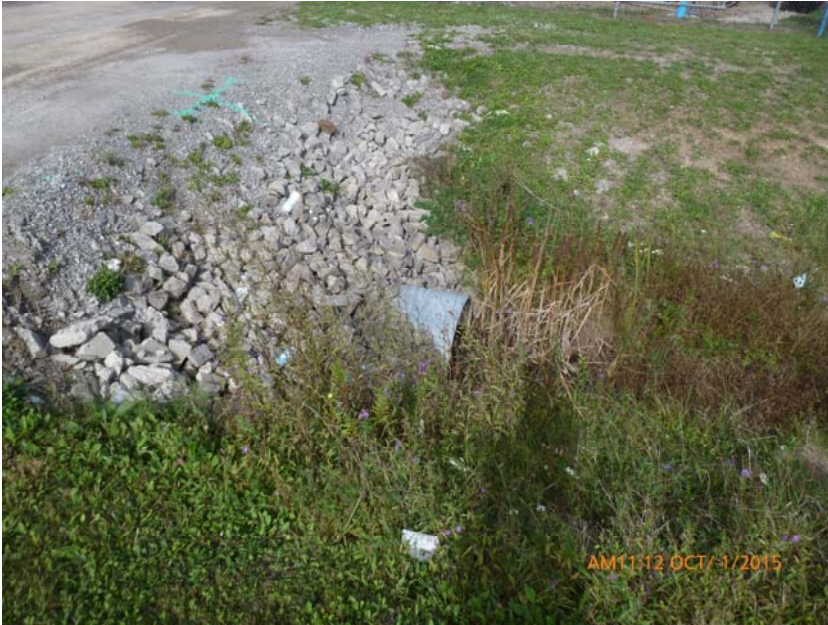
Photo 25: Driveway culvert inlet.
