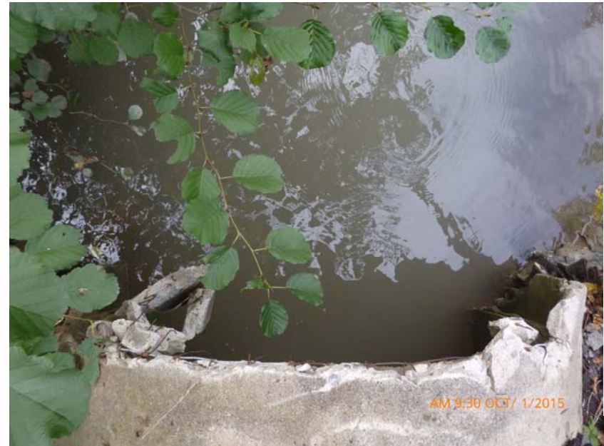
Photo 8: Culvert outlet in state of disrepair.
