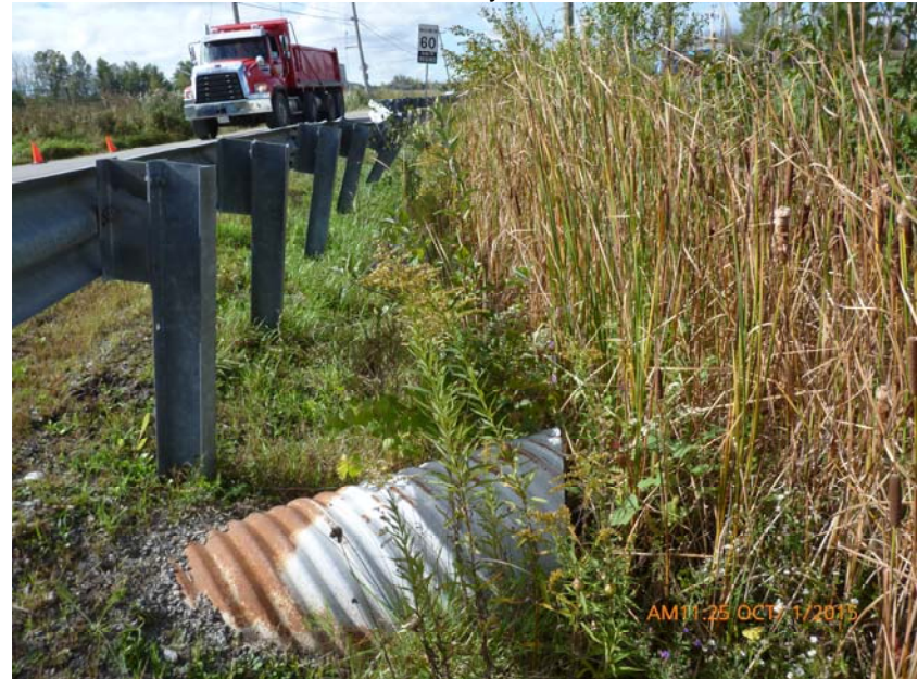
Photo 28: Culvert outlet to north ditch with thick vegetation.
