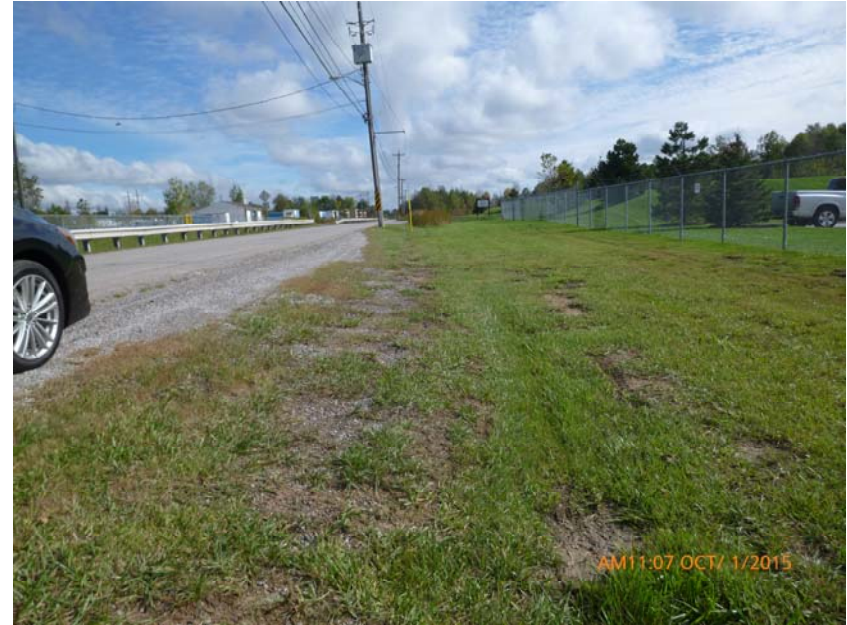
Photo 22: South ditch - shallow and regularly maintained.
