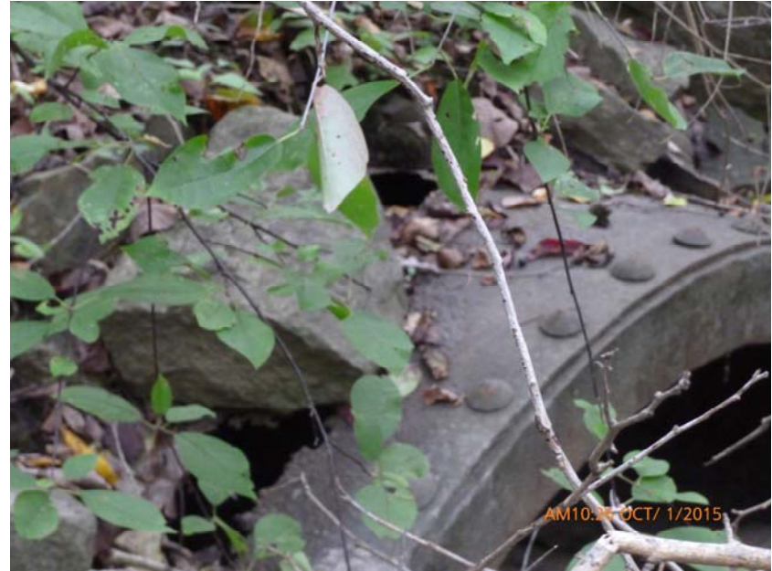
Photo 18: Culvert outlet heavily corroded with holes in the pipe wall.
