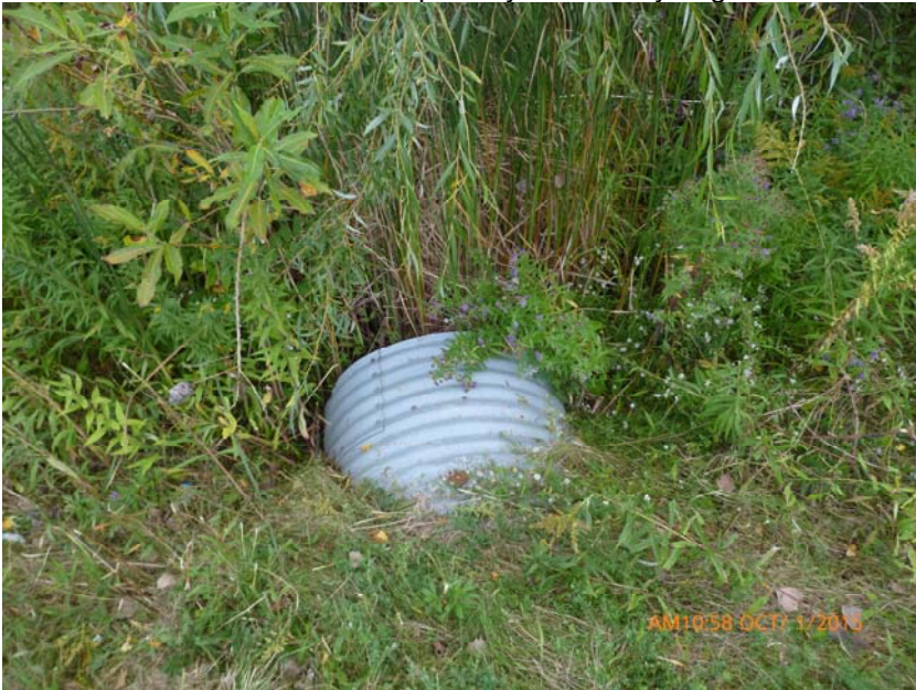
Photo 19: Culvert inlet in good condition.
