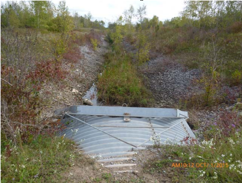
Photo 15: Conrail Drain Channel - looking upstream. Vegetation growth within channel.
