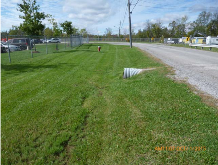
Photo 21: South ditch - with CSP culvert in good condition.
