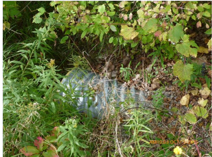
Photo 12: Culvert outlet in good condition.
